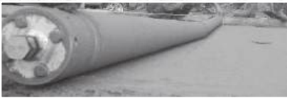
6. CV Joint - Crowned and cambered pours
