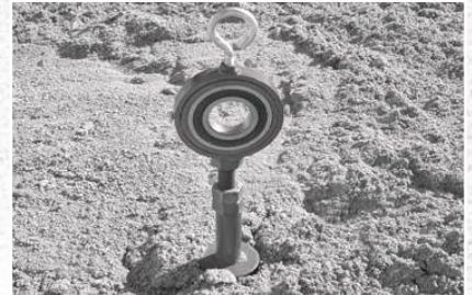
Insert pivot bearing in the tube. Use the two nuts to adjust the height for the center of the pour. The top of the pour is 3/8 inch up from the bottom edge of the pivot bearing nut. Tighten the two nuts against each other at the correct height.
